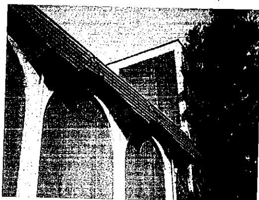
Bldg. 1200 – Trees adjacent roof line requiring trimming
